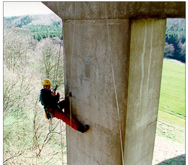
Bridge inspection using in-house roped access certified personnel
